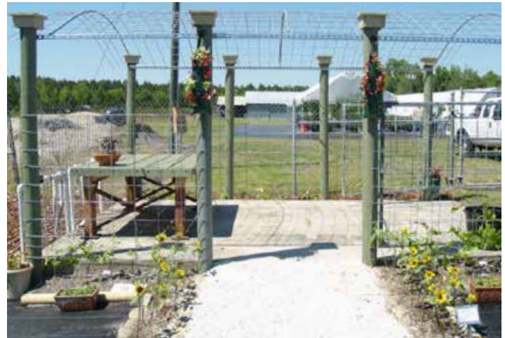
FIGURE 5. Arbor built over an existing concrete slab (Credit: Joe Sowards)
