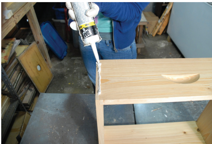
Figure 3. Caulking joints helps seal out moisture.
