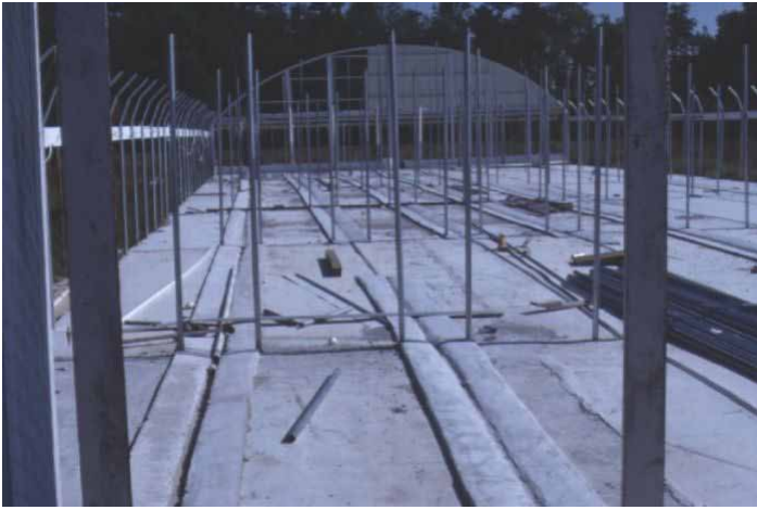
Figure 4. Construction of leachate collection system in a new greenhouse Credits: UF/IFAS
