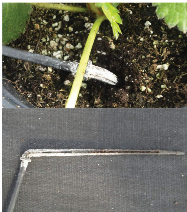
Figure 2. Scale-like deposits in a microirrigation system for peach production Credits: Guodong Liu
