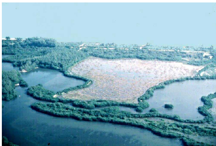
Figure 2. Vegetation damage in an overflooded impoundment.
