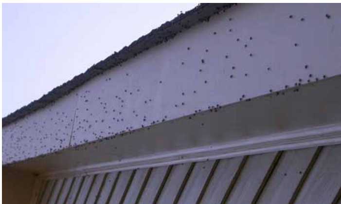
Figure 7. Infestation of adult bean plataspids, Megacopta cribraria (Fabricius), on a local house in Georgia, USA. Megacopta cribraria have an overwintering stage during their life cycle and tend to swarm to nearby buildings during the overwintering period.
