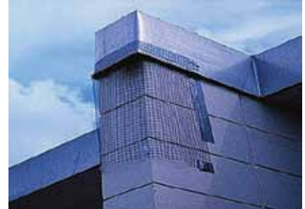
FIGURE 14 • Devices, such as bat netting, can be placed where birds or bats reside to allow one-way movement out of the cavity, thus they can also be used for exclusion.
