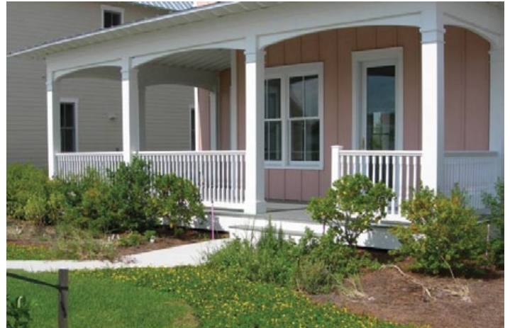
FIGURE 8. Small, fine-textured shrubs allow easy access to porch railing for maintenance.
