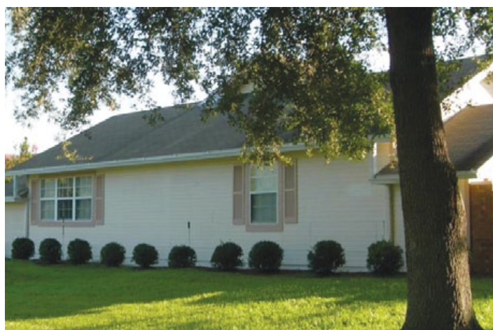
FIGURE 5. Shrubs along wall are overtrimmed.
