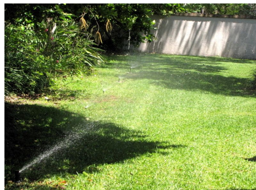
Figure 2. Mixed sprinkler types. Note: rotary sprinkler in foreground and spray heads in background (photo by Bernard Cardenas).
