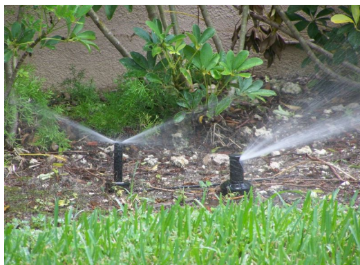
Figure 1. Ornaments and turfgrass being irrigated from the same irrigation zone. Note: the spray head in the background is irrigating the ornaments and the rotary sprinkler is irrigating the turfgrass in the foreground (photo by Michael Gutierrez).
