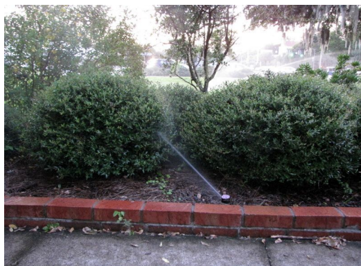
Figure 3. Blocked water spray (photo by Bernard Cardenas).
