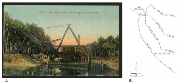
Figure 3. A) The dredge Everglade, draining the Everglades, Florida. Palatka, Fla., ca. 1910. B) Four muck-scaped canals that dissected the Everglades by 1917 (Light and Dineen 1994).
