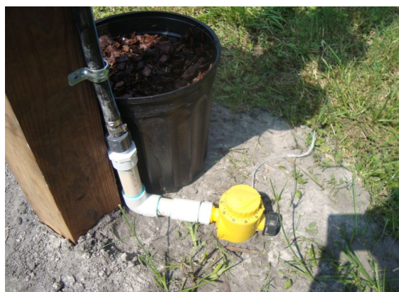
Figure 9. Install water timer (optional). (Credit: B. M. Santos and T. P. Salame-Donoso)
