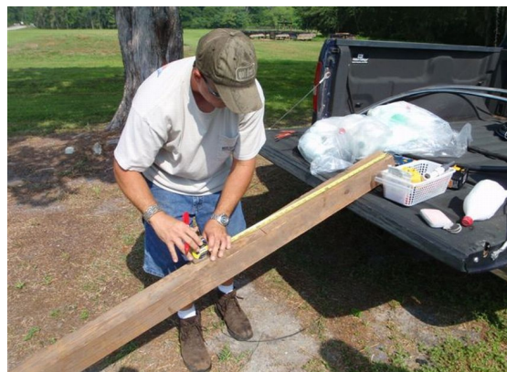
Figure 3. Measure the underground 2 ft of the pole. (Credit: B. M. Santos and T. P. Salame-Donoso)
