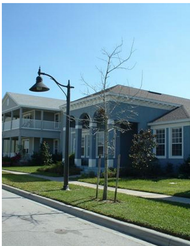
Figure 1. Full cutoff street lights installed along transportation routes in Harmony, FL. Credits: Photo: Jennifer Van Walford
