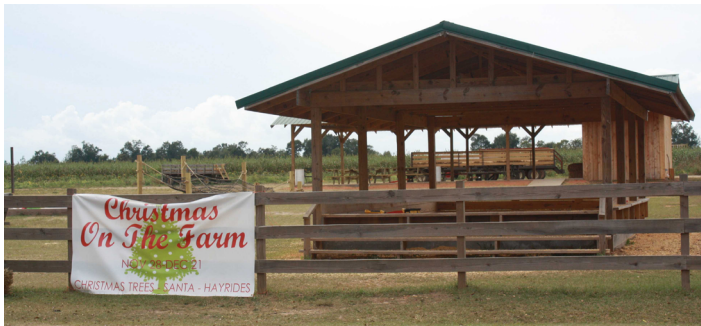
Figure 1. Nonresidential farm building. Credits: M. E. Henry, UF/IFAS
