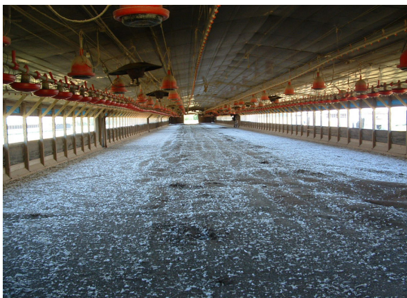
Figure 1. Typical broiler poultry house ready for clean-out. Credits: G. Hochmut
