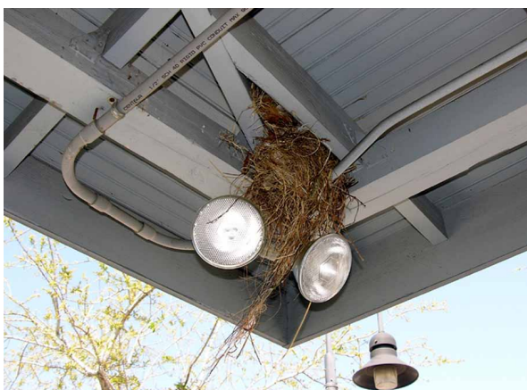
Figure 9. House Sparrows build messy nests of dried vegetation in any available space on urban structures—under eaves, above and behind gutters and drainpipes, in and around vents, and especially around signs. These nests should be prevented or removed because they can cause fire hazards and clog drains, and the droppings that accumulate under the nests can present a health hazard and cause unsightly stains. Credits: Steve A. Johnson, University of Florida, 2008
