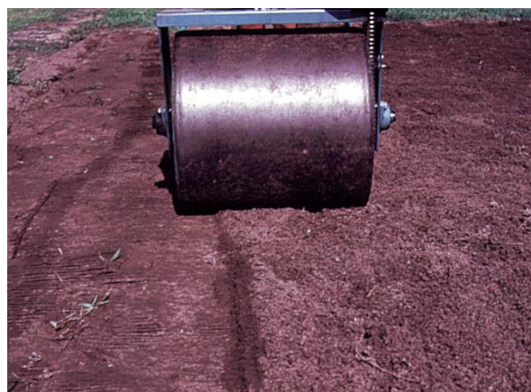
Figure 2. Final Grading
