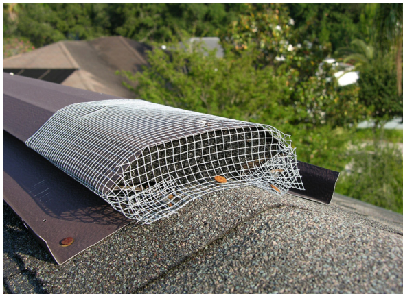
Figure 9. Openings that allow access to attics, eaves, or other potential nesting sites for European Starlings should be securely covered. Here, hardware cloth and nails are used to cover a roof vent to prevent wildlife from gaining access to the attic. Credits: Steve A. Johnson, University of Florida, 2007
