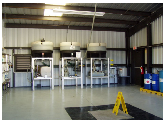
Figure 8. Bulk storage tanks holding spray mix and rinse for later use. Credits: F.M. Fishel, UF/IFAS PIO.
