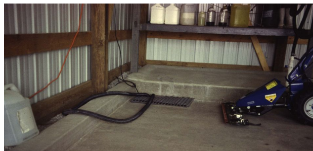
Figure 5. Permanent concrete mixing and loading area with diked edging for containment. Credits: F.M. Fishel, UF/IFAS PIO.
