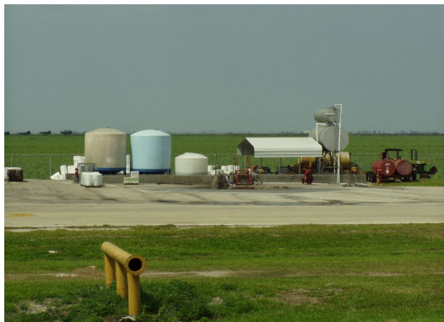
Figure 7. Bulk storage tanks on diked-concrete pad. Credits: F.M. Fishel, UF/IFAS PIO.
