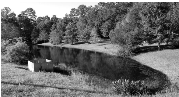
Figure 1. Retention ponds help remove pollutants from storm water. Credits: Photo by: Larry Korhnak
