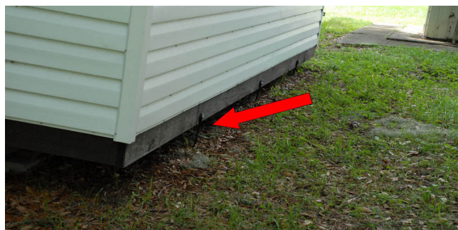
Figure 12. Opening under shed.
