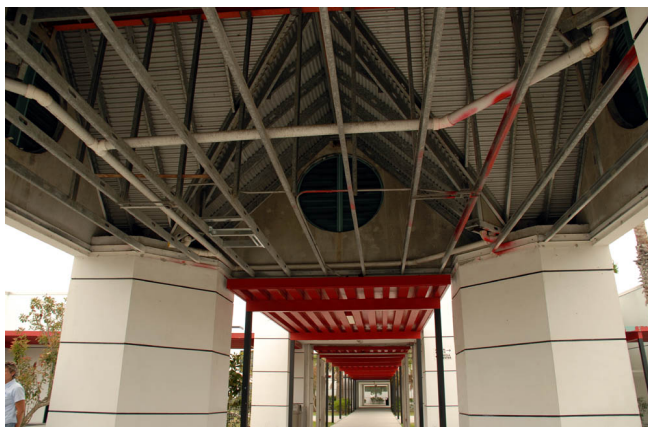
Figure 7. Large recess under roof.
