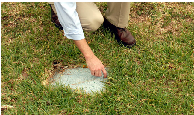
Figure 1. Closed water meter.
