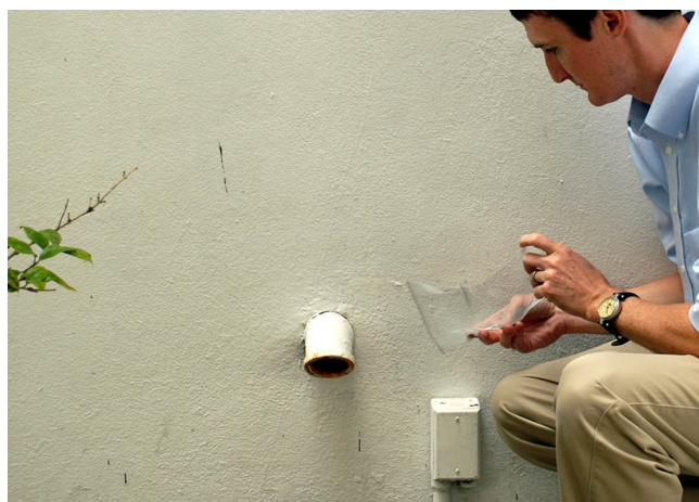
Figure 19. Placing screening over pipe.
