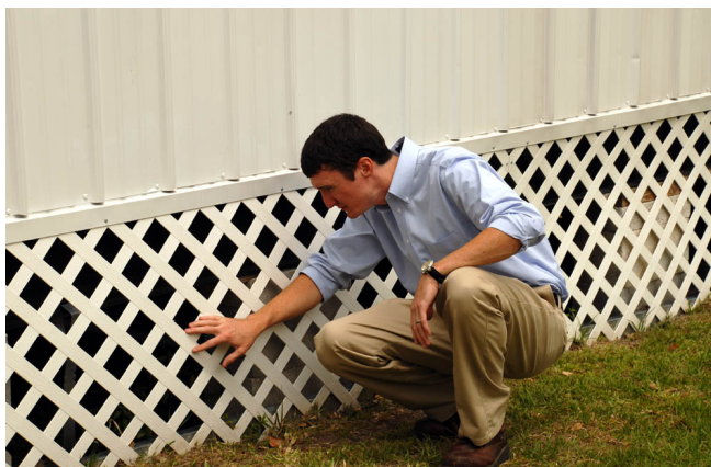
Figure 8. Inspecting under house.
