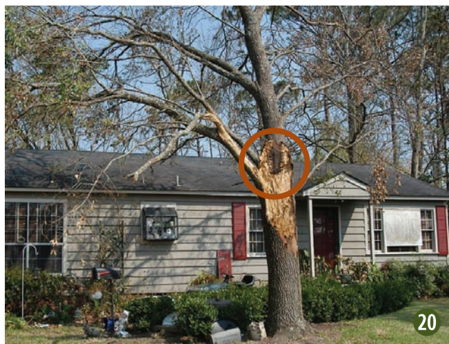
Figure 20 Notice the the dark area at the top of the split: it is a bark inclusion. The stem broke in Hurricane Katrina at this point of weak attachment.
