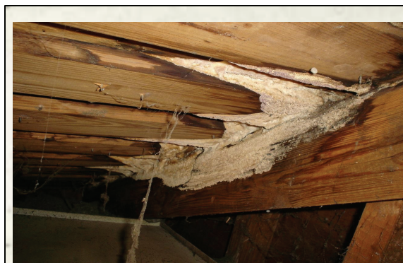
Massive amounts of mold infect local business' attic. This amount of mold growth could cause serious health problems for employees and patrons.
