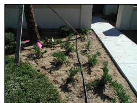
Figure 3. Microspray or microjets in a plant bed. Photo - Michael Dukes Credits: Photo - Michael Dukes
