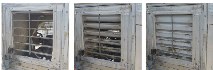
Figure 6. Ventilation and cooling fans should be equipped with anti-back draft shutters as shown here from left to right in the open, partially opened, and closed positions.
