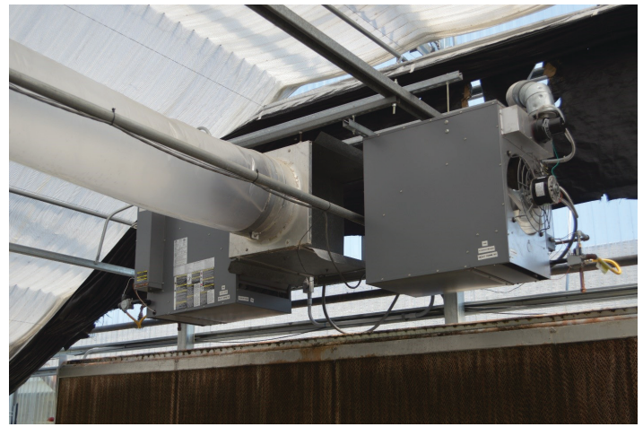
Figure 3. Fan-jet poly-tube system with heaters.
