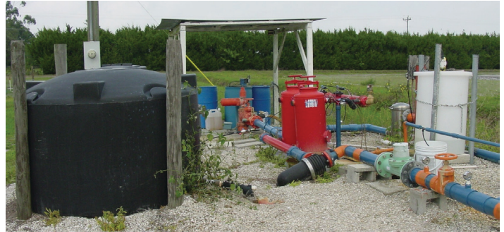
Figure 2. Fertigation equipment, including fertilizer tank (left), filters (center), and injector (right). Credits: Mongi Zekri, UF/IFAS
