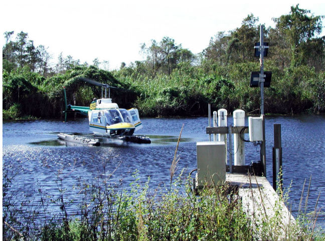
Figure 2. A completed water quality monitoring station.
