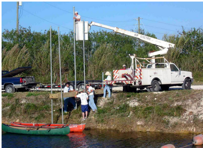
Figure 1. Site selection and construction.
