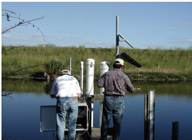
Figure 10. Site visit and routine maintenance.
