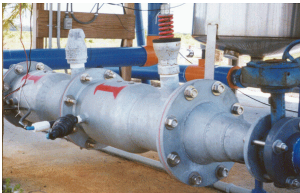
Figure 1. Typical backflow prevention device with vacuum breaker, check valve, and low pressure drain.
