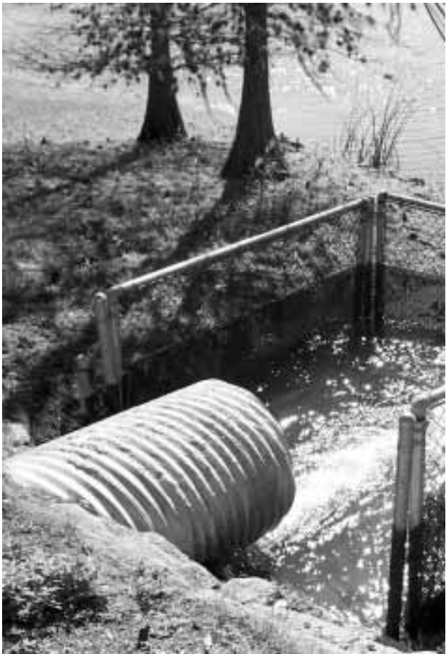
City of Orlando Streets, Drainage and Stormwater Utility
