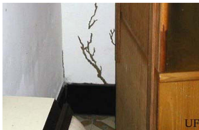
Figure 4. Soil tubes of the Formosan subterranean termite, Coptotermes formosanus Shiraki. Credits: Nan-Yao Su, University of Florida
