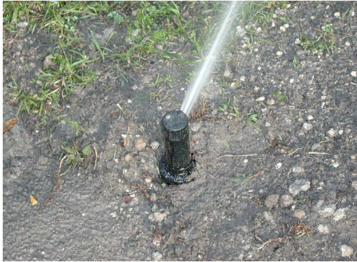
Figure 6. Type of traditional landscape and turf irrigation emission devices: Gear-driven rotor sprinkler.
