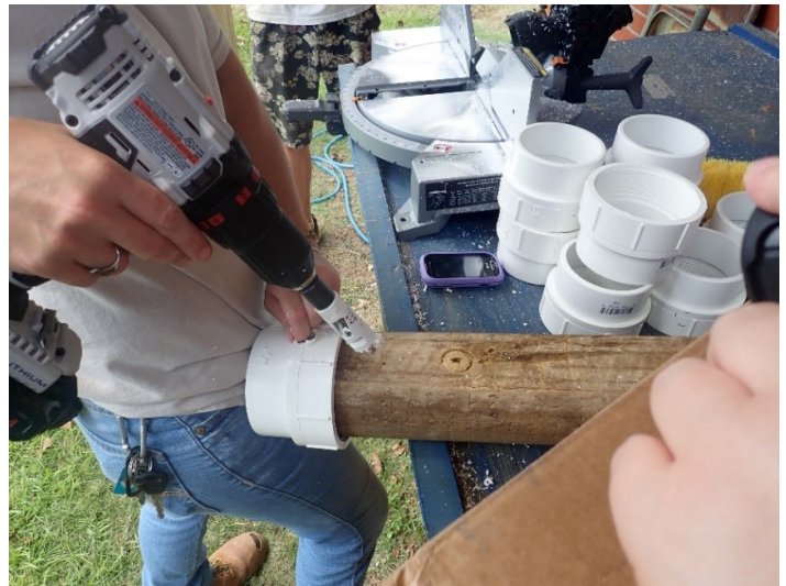
Figure 12. A 4-inch PVC slip thread adapter is drilled on the side using a hole saw (1 1/8-inch diameter) for the bottom of the siphon.
