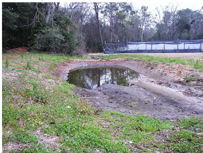
Figure 2. Basin installed downstream from wooden boards.
