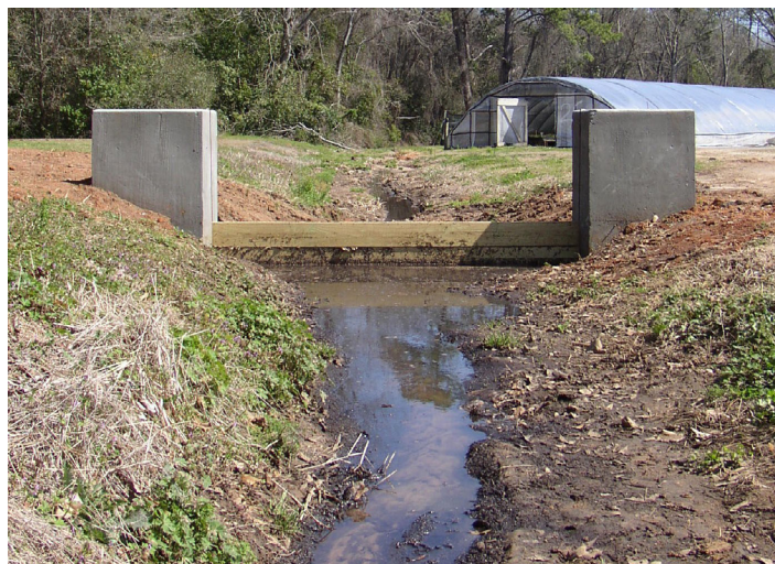
Figure 1. Wooden boards installed for management of runoff from watering station located upstream.
