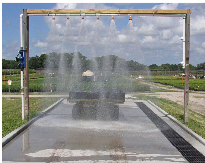
Figure 3. Concrete pad installed for runoff management at the watering station.
