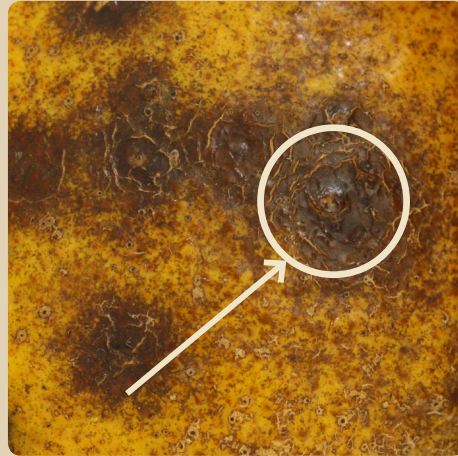
Close view of cracked spot with hard spots forming
