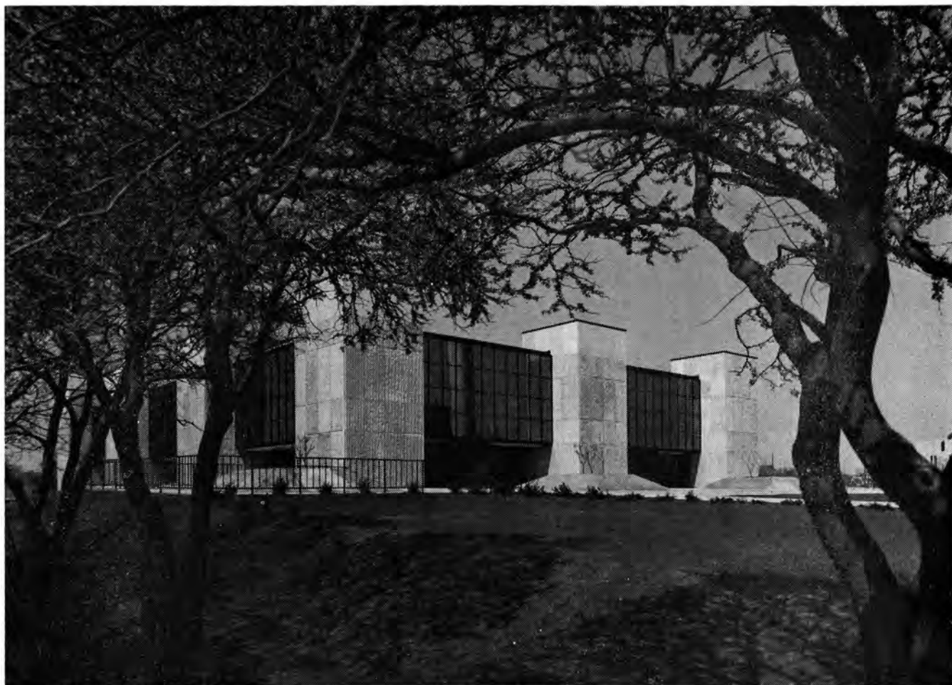
DURLAND HALL—New Home of Chemical Engineering
