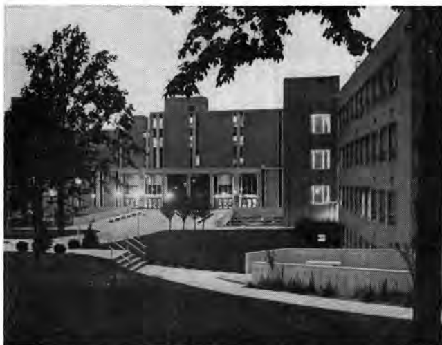
AUBURN SCIENCE AND ENGINEERING CENTER
