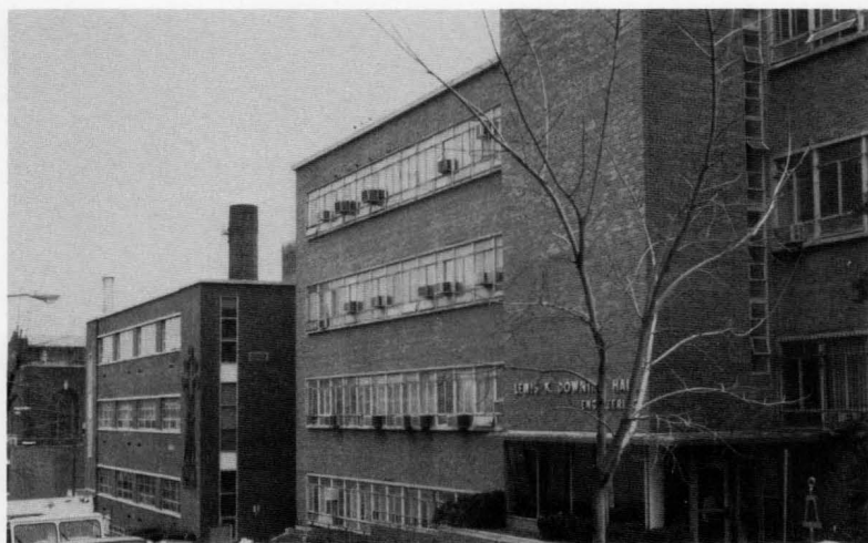
Downing Hall of Engineering: Chemical Engineering Wing on the left.
