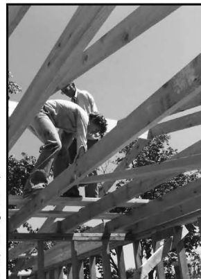
▶ Hands-on house construction of parent's house in Carbondale, 1978.
