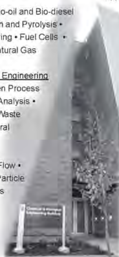
The new CHBE building, opened in March 2006, houses world-class research and teaching activities. The top 2 floors are dedicated to graduate student offices and research labs - electrochemical, fuel cell, thermodynamics, polymer rheology, biomedical research, imaging and sensor development and fine particle, mixing and water treatment, bioprocessing, etc.
