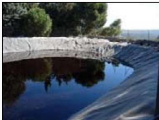
**Figure 1.** Artificial lagoons are used for storage and natural evaporation of olive mill wastewater.
