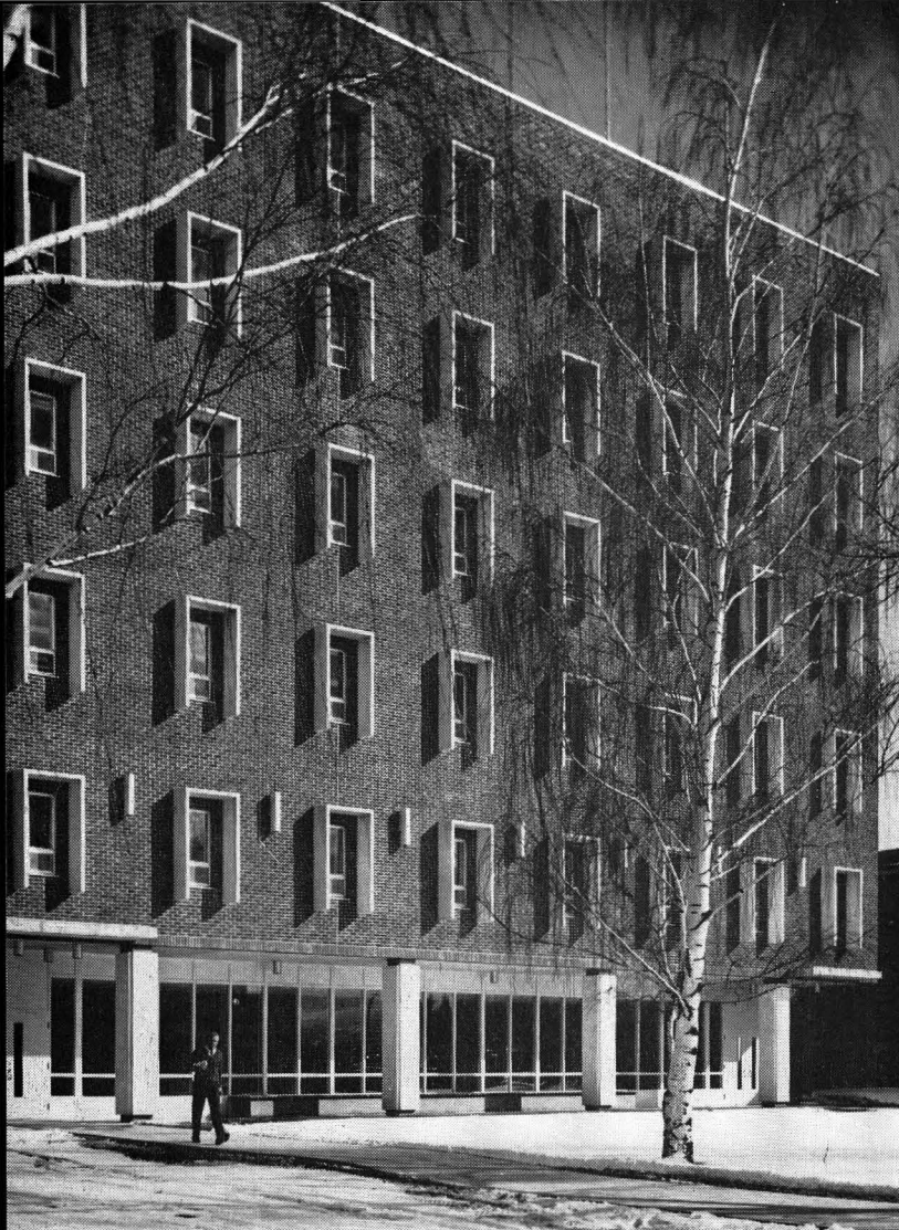
Cobleigh Hall: ChE occupies the 3rd and 4th floors.
