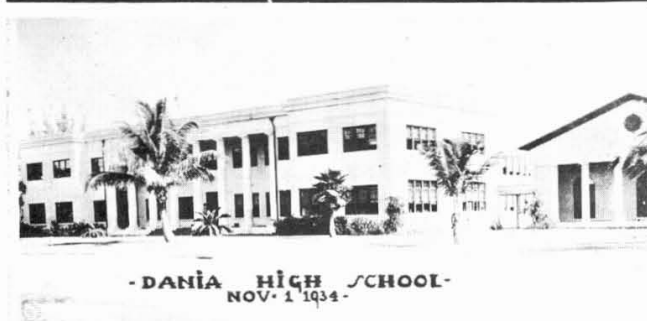
Plans are underway to rehabilitate Dania School for use as a community center. This photograph appears courtesy of Mrs. Lillian McMillan.
