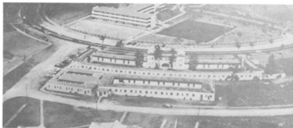
Riverside Military Academy, c. 1967. By this time the old Hollywood Hills Inn in the center of the circle had been replaced by a new barracks building.
