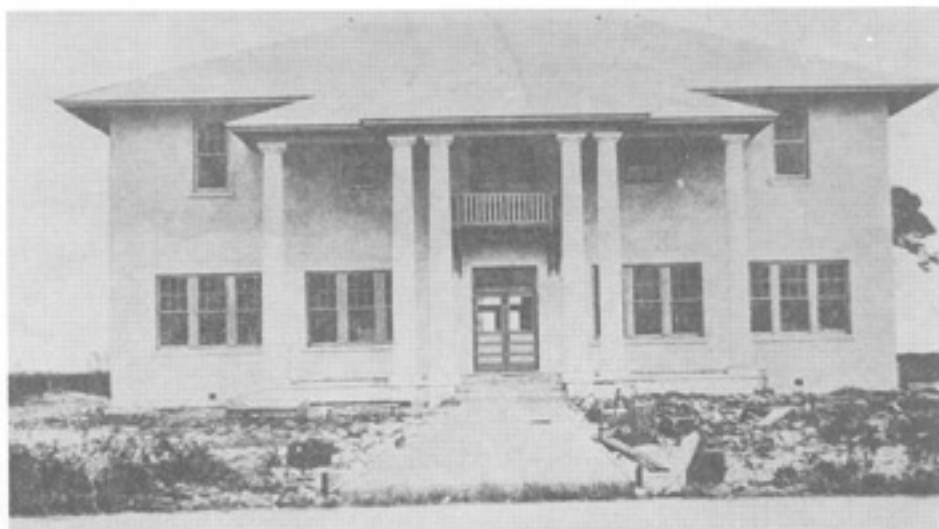
The Dania school building soon after completion in 1913. Note construction debris still on the ground.
