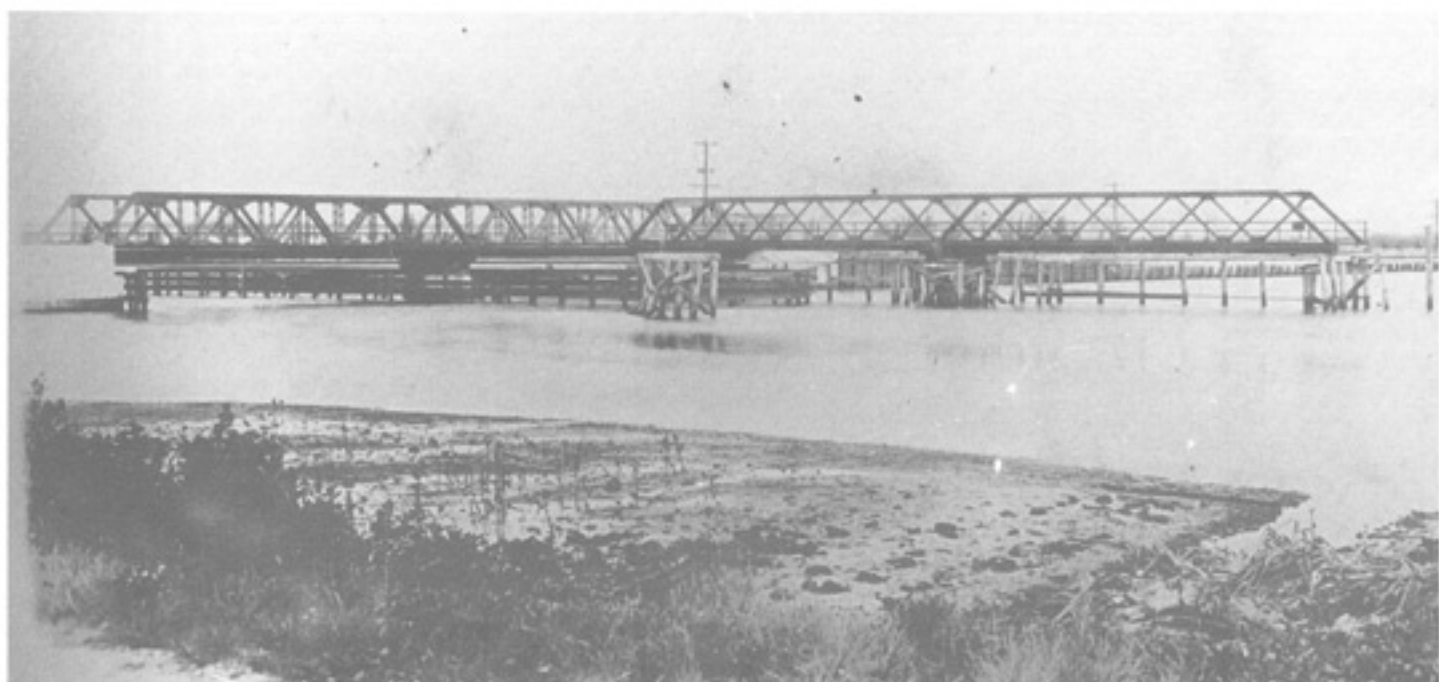
Removal of the old turnstile bridge (right) over the Intracoastal at Las Olas Boulevard, and installation of the new bridge (left), 1925. The old bridge was moved to Oakland Park Boulevard (photo courtesy of Fort Lauderdale Historical Society).
