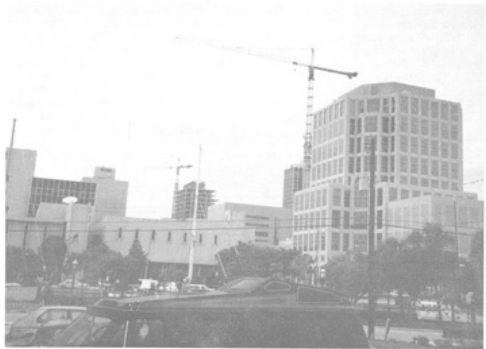
Downtown Fort Lauderdale's skyline, 1990, showing numerous construction projects underway.
