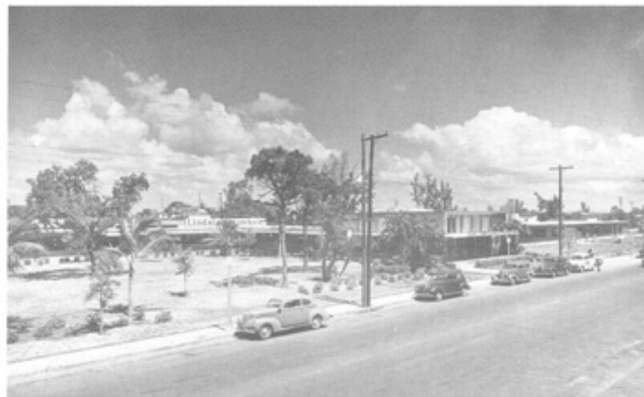
The Fort Lauderdale City Hall on North Andrews Avenue, shortly after its 1948 completion.
