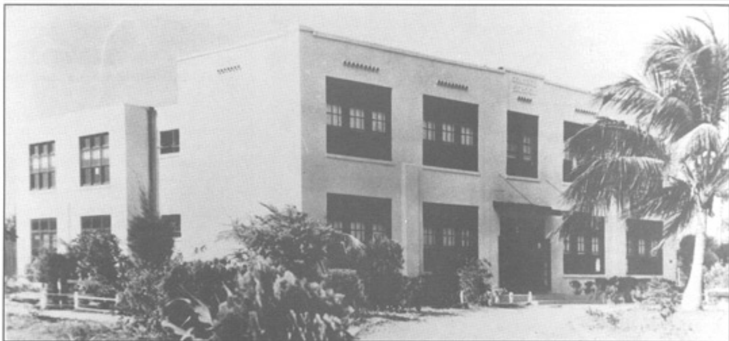
The Old Dillard School, 1001 Northwest Fourth Street, Fort Lauderdale, 1942.
