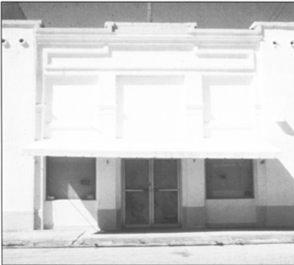
Bank of Pompano, built 1922 61 NE 1 st Street, Pompano Beach This combination Mediterranean Revival and Neo-Classical style building could meet the criteria for listing in the National Register.
