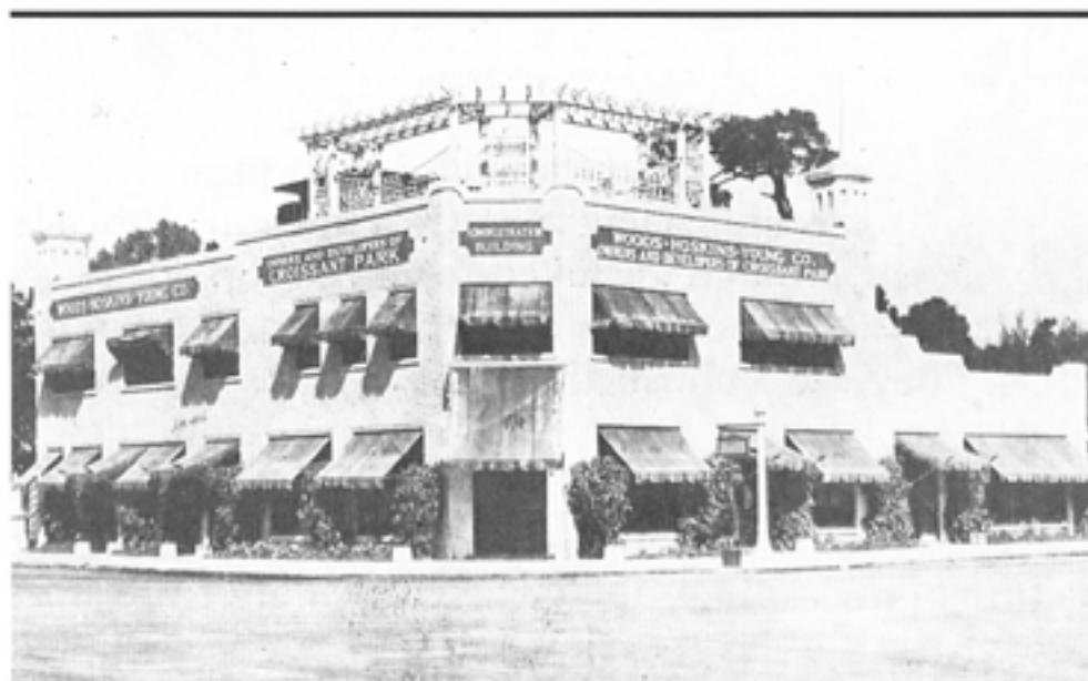
CROISSANT PARK ADMINISTRATION BUILDING, circa 1926 (From Croissant Park Pictures Before and After the Storm of September 18, 1926 , Woods-Hoskins-Young Company brochure)
