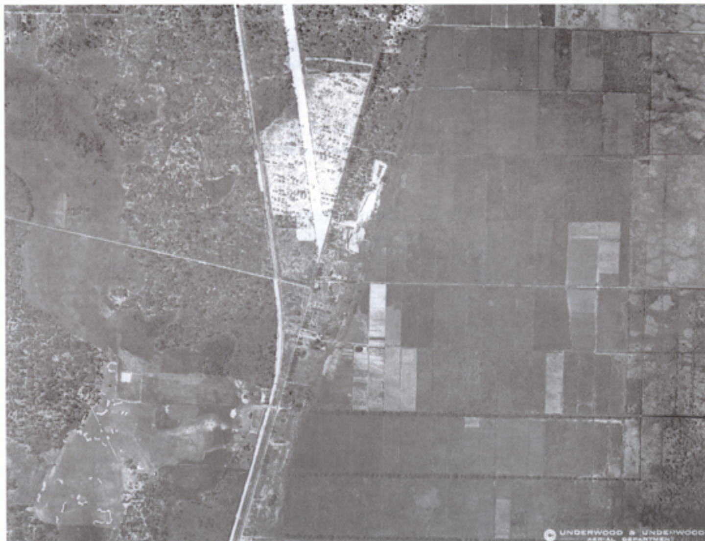
1925 view, looking north toward the newly-extended Andrews Avenue, of the South Side Golf Course, future site of Fort Lauderdale-Hollywood International Airport.
