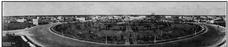
Fig. 14. Detail from a panoramic image looking west across Circle Park to Hollywood Boulevard. The Great Southern Hotel is the building on the left, clearly showing the two ends of the U joined by a single-story connector that appears to have been enclosed, possibly a dining room. The image is dated Oct. 27, 1927. (Courtesy of the Hollywood Historical Society.)
